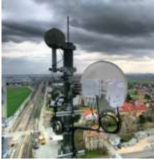
Exhibit 6: Dual band antenna
